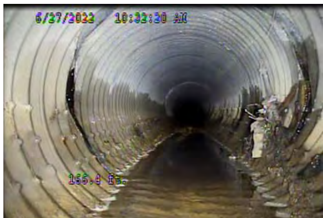
Photo 2: Debris in pipe
