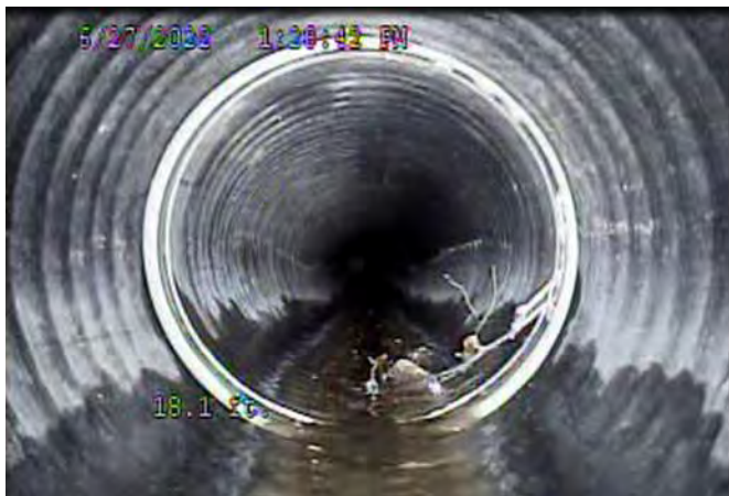
Photo 1: Separated joint & debris
