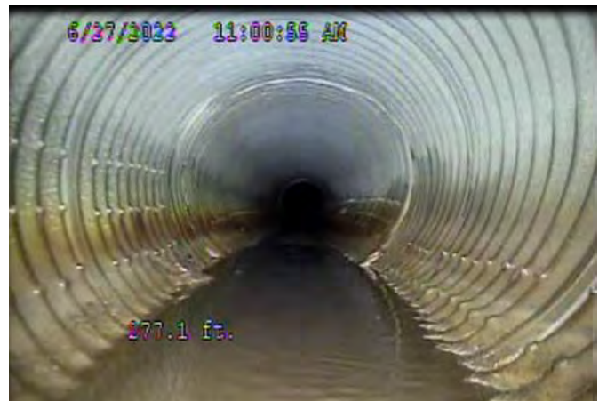
Photo 2: Belly in pipe
