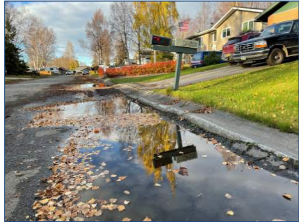
Existing Ponding and Heaved, Irregular Curbs
