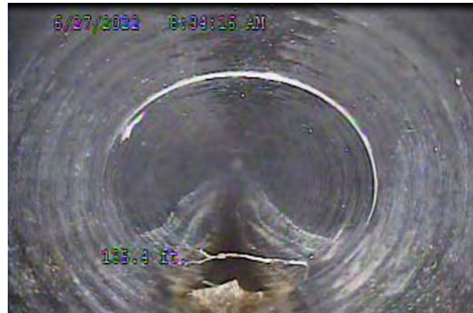
Photo 2: Debris and pipe ovality
