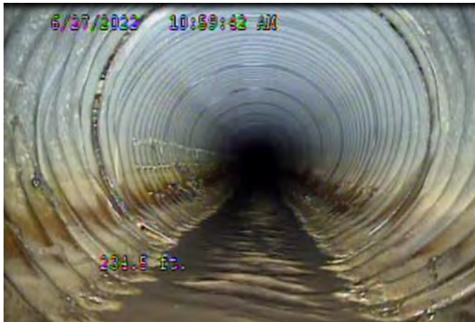
Photo 1: Separated pipe joint
