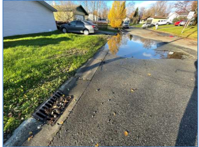
Ineffective Catch Basin / Ponding Upstream
