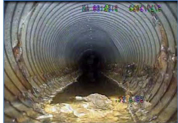
Photo 2 - Pipe 28650 (Mineral Deposit at Pipe Joint)
