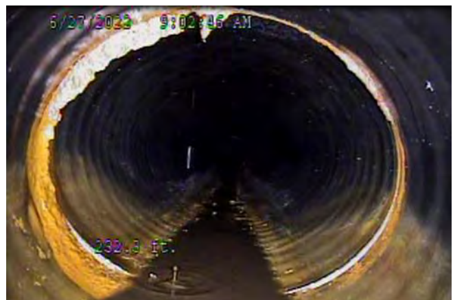
Photo 2: Infiltration/mineralization and belly at pipe joint
