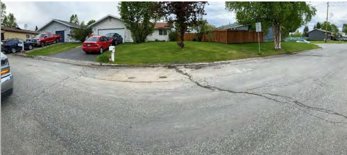
06/02/2021: BH-01 and BH-01 redrill (second attempt at 15-foot sample) after completion. BH-01 (left) backfilled with cuttings and cold patched. BH-01 redrill (right) completed as piezometer with flush mount steel monument.
