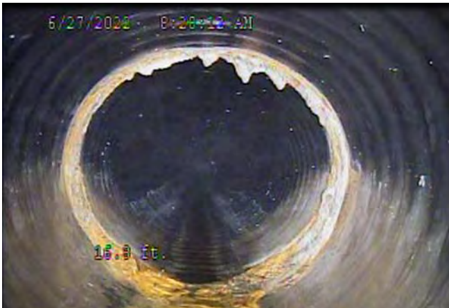
Photo 1: Infiltration/mineralization
