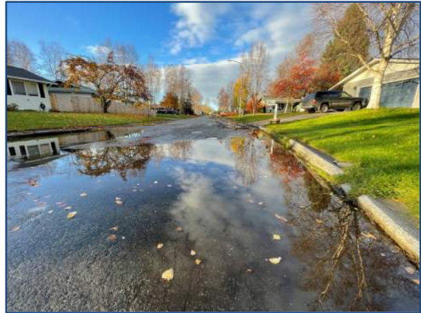
Ponding and Heaving Curb & Gutter
