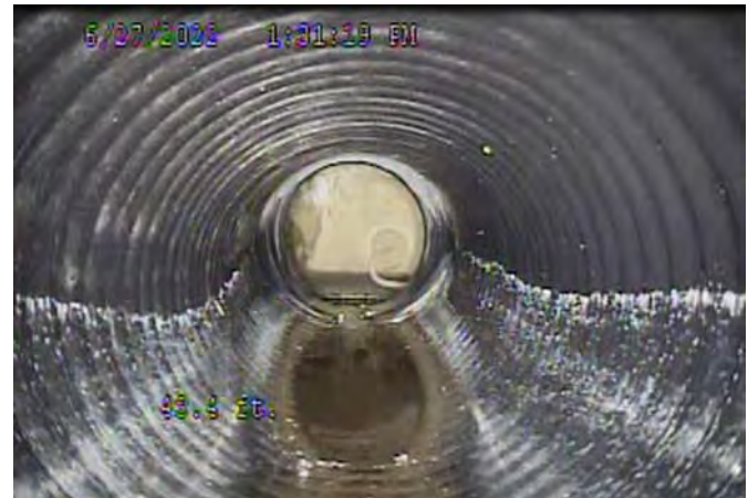
Photo 2: Belly/low point in pipe
