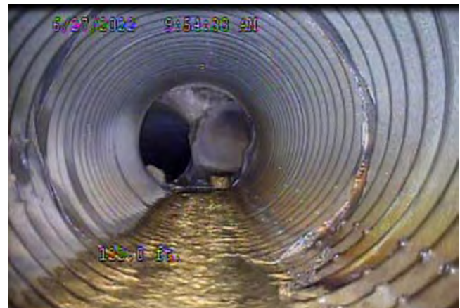
Photo 2: Separated pipe joint
