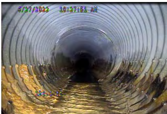
Photo 1: Infiltration/mineralization through perforations
