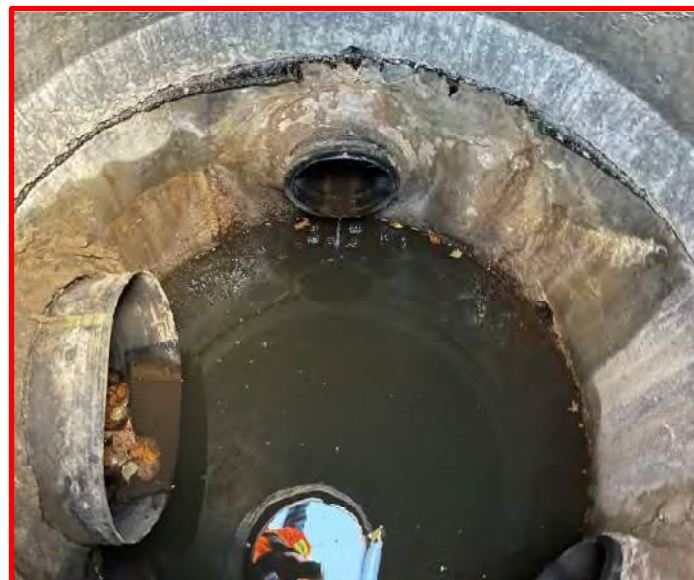
Photo 6 - Infiltration at Base/Cone Joint
