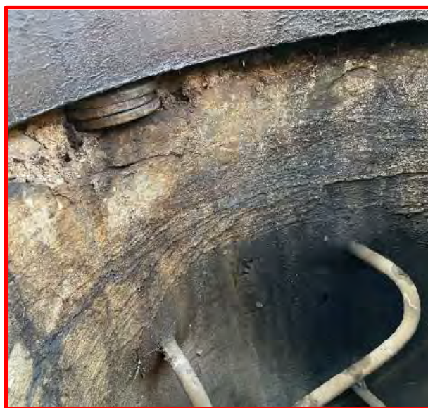
Photo 5 - Metal Shims/Spacers in Grade Ring
